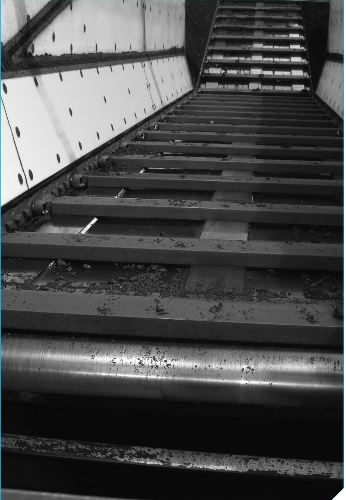
Feeder Breaker Ketting
